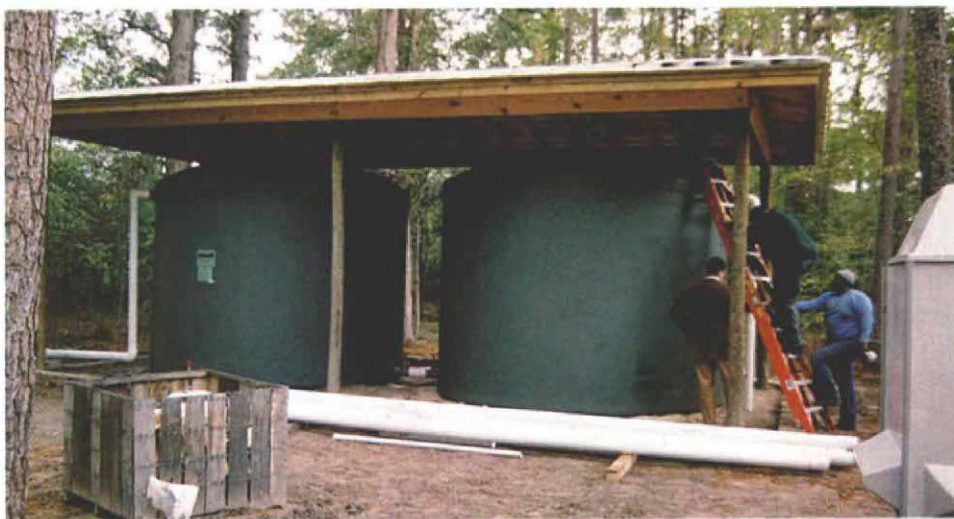
Aboveground tanks need a roof. Fiberglass tanks installed aboveground can be used for water storage, but a roof is needed to keep fiberglass from breaking down in the sunlight. Water does not stay as cool as with in-ground tanks.
